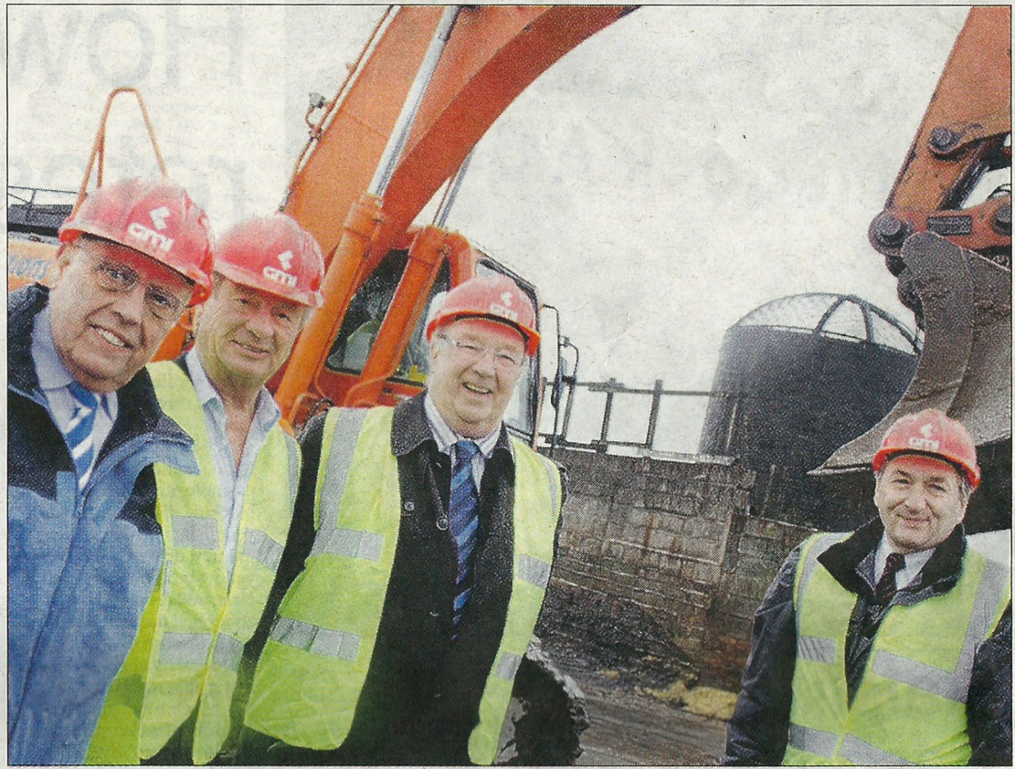
● Work starts: Cllr Graham Baxter, leader of North East Derbyshire District Council; Peter Gilman, chairman of the GMI Group of companies; Cllr David Nuttall, former North East Derbyshire District Council leader and Clay Cross member – who led the launch of the Clay Cross regeneration project – and Cllr Peter Riggott, NEDDC's member champion for the regeneration scheme.
